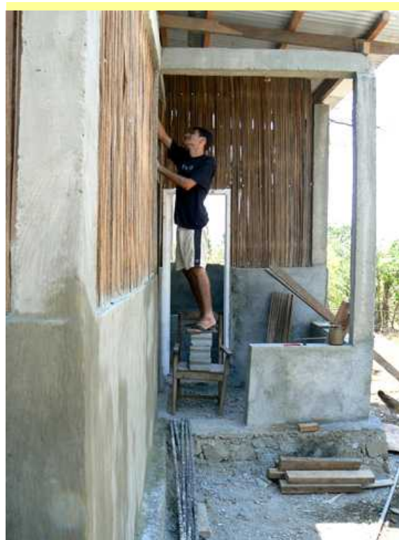
Painting a House in Liquiça
